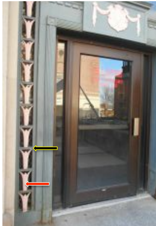
Figure A4. Contemporary view of north elevation doorway showing doorframe grill (see black arrow) with palmette ornaments (see red arrow).
