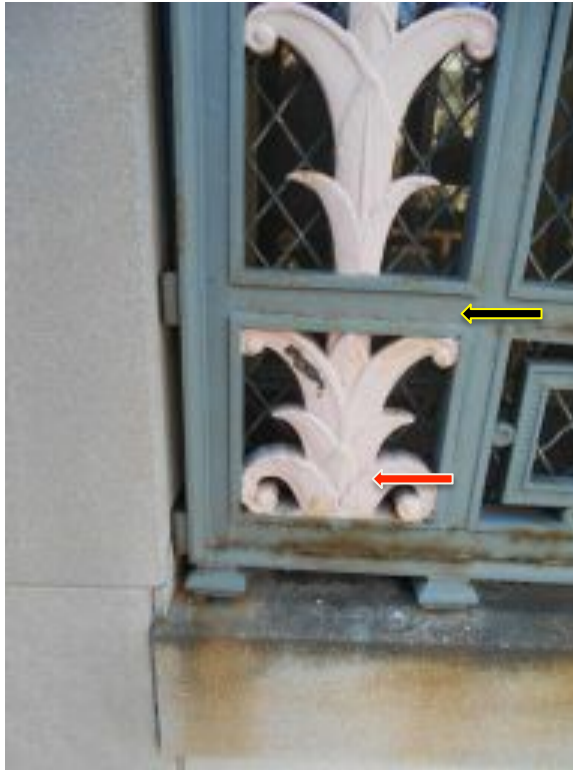
Figure A7. Contemporary view of north elevation vertical grill frame (see black arrow) and anthemion ornament elements (see red arrow).
