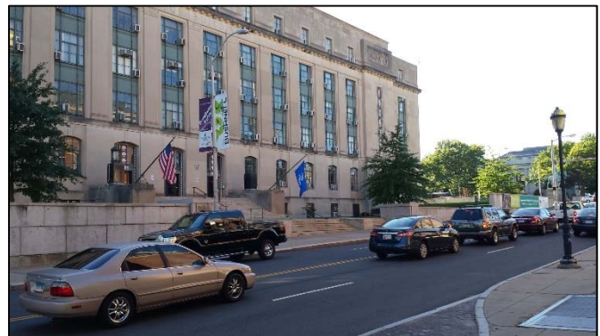
SOB from Capitol Avenue
