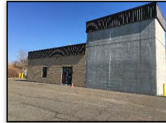
Return Sludge Building
