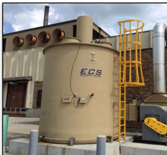
FIGURE 6-3 TYPICAL ACTIVATED CARBON SYSTEM
