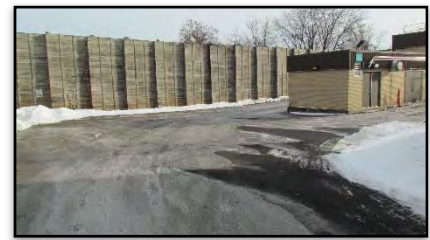
Spill Containment Area
