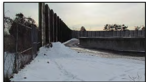
Final Settling Tank Access
