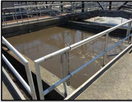
Zone A Walls
