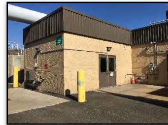
Septage Receiving Building
