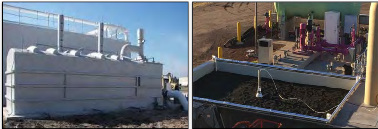
FIGURE 6-2 TYPICAL PACKAGED BIOFILTER
