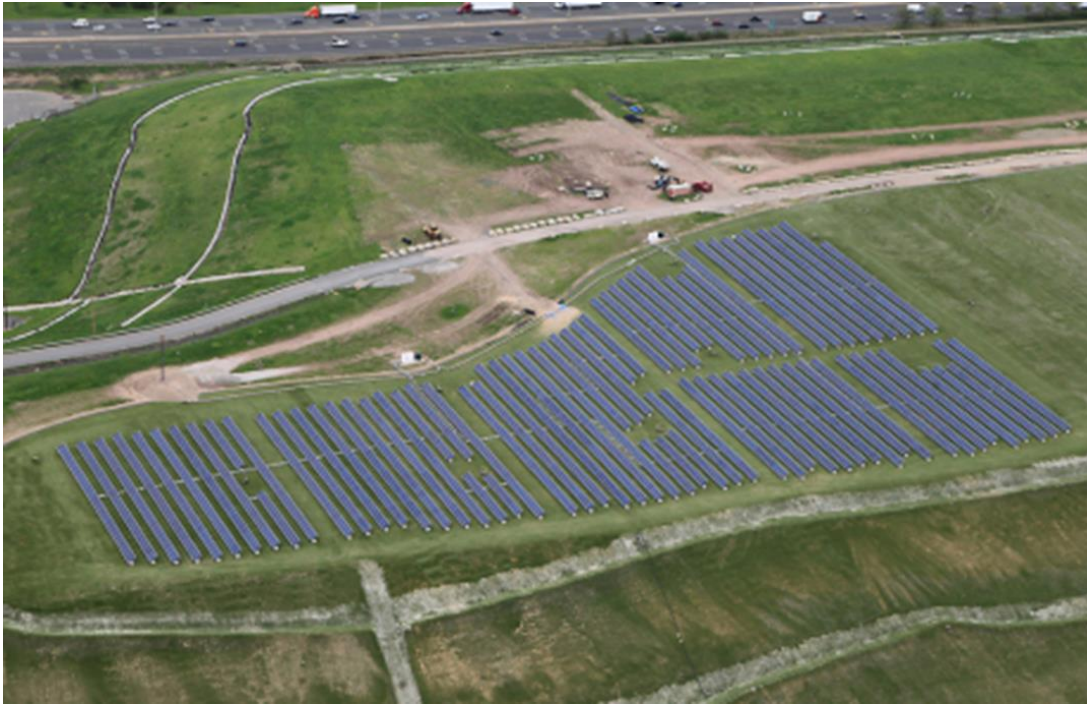
The Hartford Landfill 1 MW solar array started production in 2014
