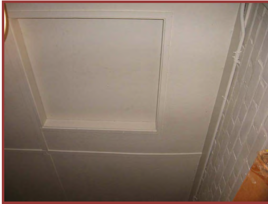
Photo 7 - View of ceiling hatch in Room 2 used to access crawl space.
