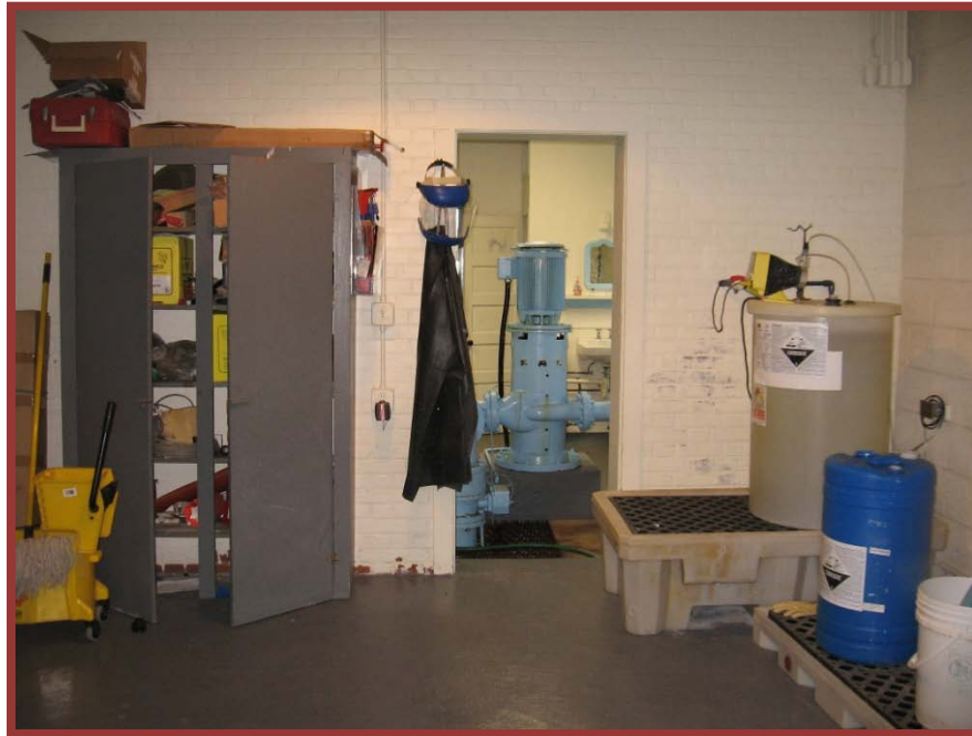
Photo 5 - View of Room 2 of Pump Station, facing north.
