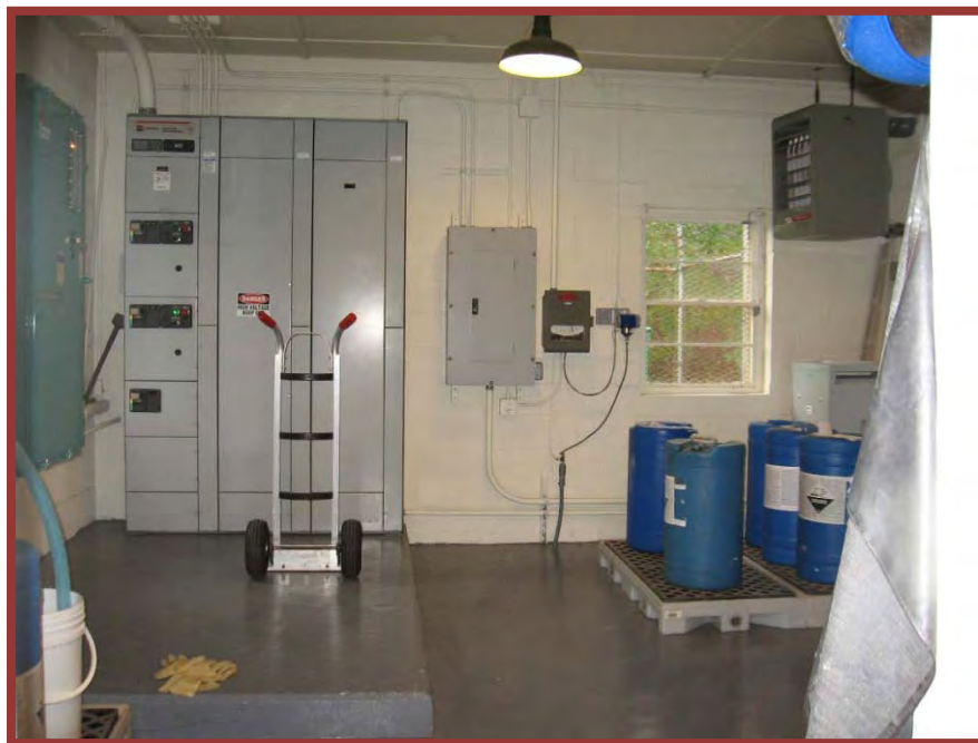
Photo 6 - View of Room 2 of Pump Station, facing south.
