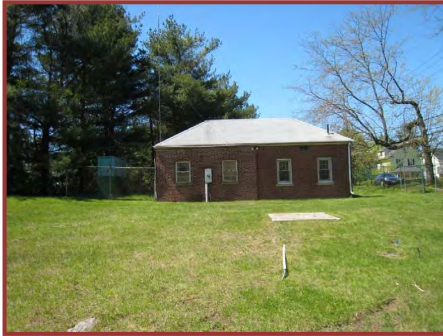
Photo 1 – View of Pump Station facing west.
