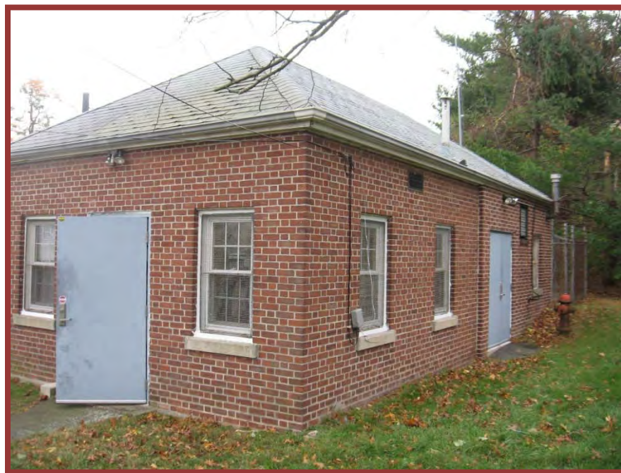
Photo 2 - View Pump Station facing south.
