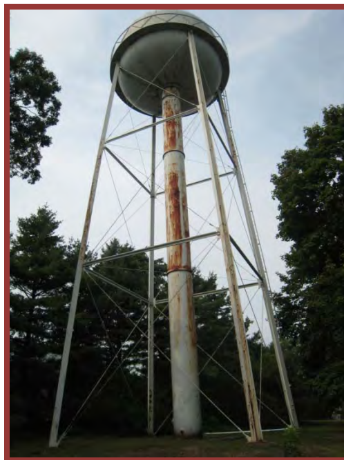
Photo 8 - View of elevated Water Tank facing north.
