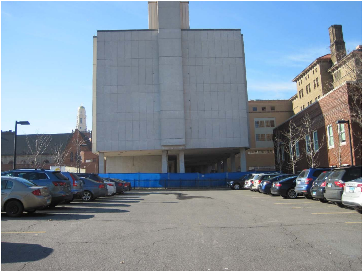
Rear of Department of Public Health Laboratory- Looking west from West Street.
