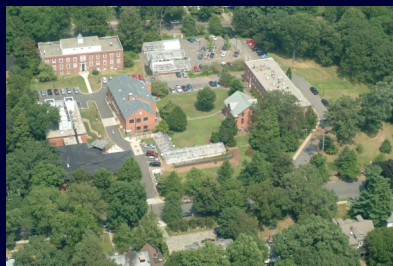
Main Laboratories, New Haven
