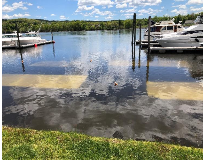
Benthic barriers installed at Portland Boat Works.
