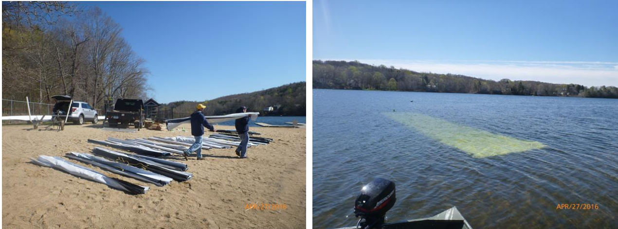
Figure 14. Benthic barrier being installed in Lake Quonnipaug, Guilford, Connecticut.
