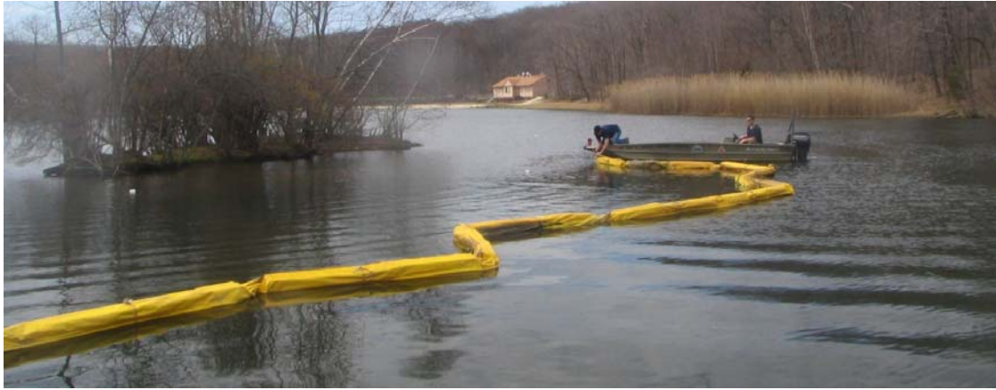
Figure 3. Installation of limnobarrier around island in Crystal Lake.
