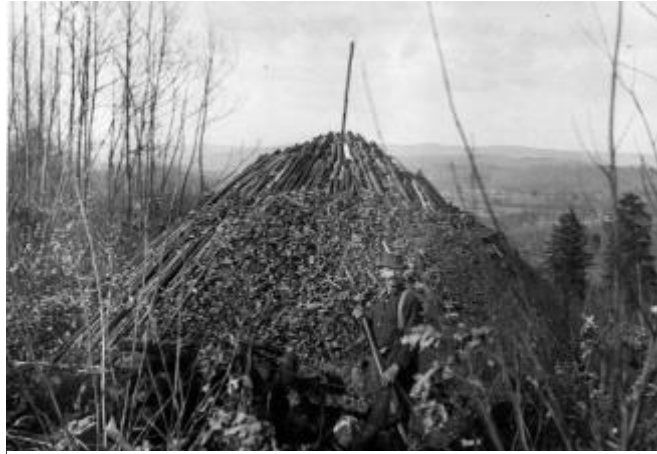
Figure 41. Charcoal pile ready was firing in Burlington, CT circa 1913 (CAES archives).
