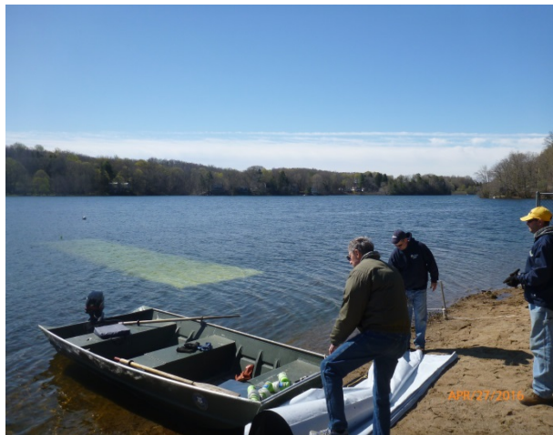
Figure 5. Installation of benthic barrier at Lake Quonnipaug, Guilford.
