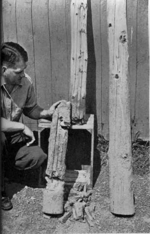
A. R. Olson of the Forestry Department examines a post destroyed by wood-rotting fungi. Post at right, in service for the same number of years, had been treated with preservative and escaped decay.
