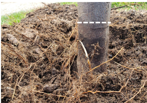
Figure 5. Incorrect application of mulch. Too thick a layer of mulch causes superficial rooting, formation of girdling roots, and exposes the bark to rot. The dashed line shows the top of the mulch layer which was 6 inches thick.
