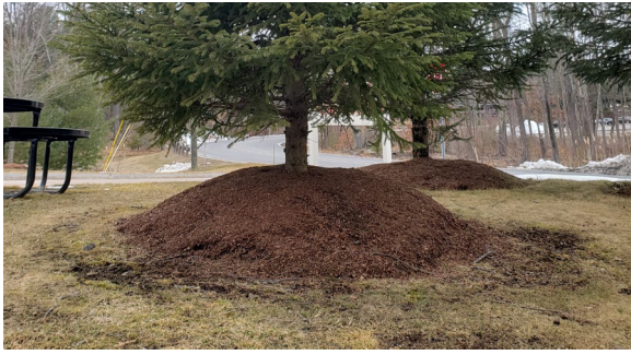
Figure 4. Incorrect application of mulch. Piling mulch at the base of the tree (“volcano mulching”) exposes the bark to rot.
