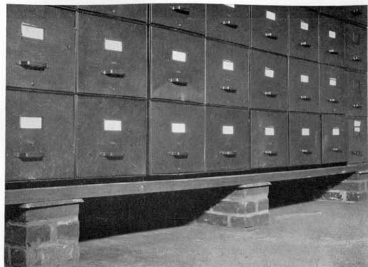
Figure 6. Records stored on a termite-proof rack in the basement of an infested building.
