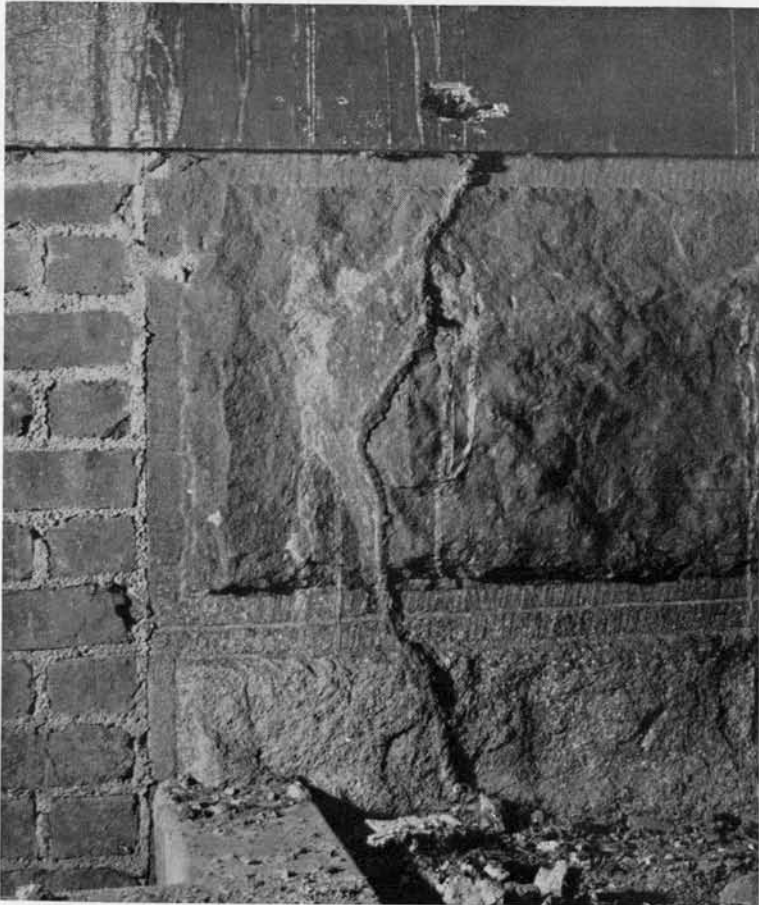
Figure 2. Termites constructed this shelter tube from wood to the ground in a partly excavated area, formerly an exterior wall.
