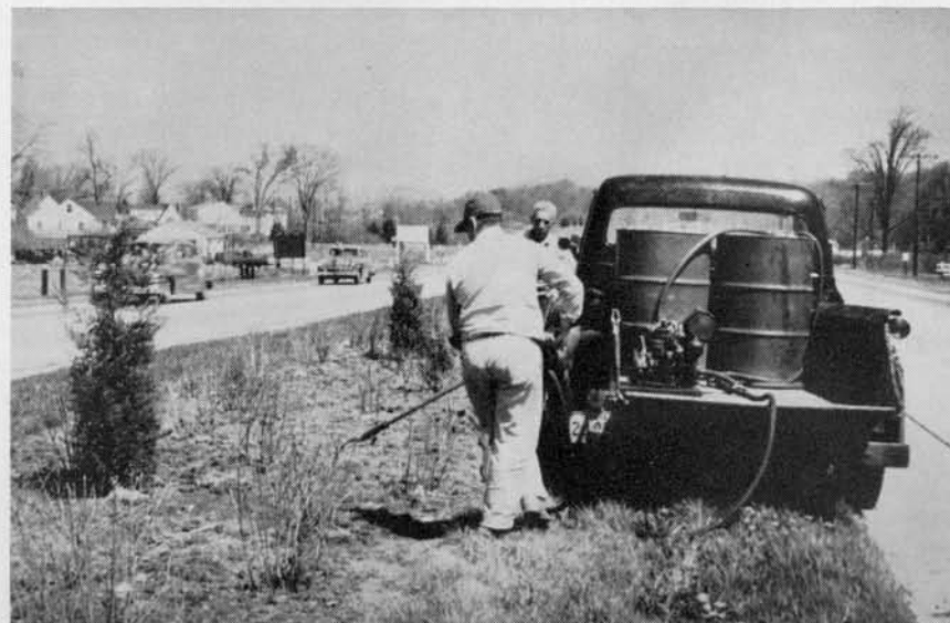
Figure 2. Hand booms from truck-mounted power spray equipment, as shown above, are often used for applying herbicides in functional plantings. They can also be used for application of basal sprays and stump treatments for brush control, and spot treatments for the control of poison ivy and other plant pests.
