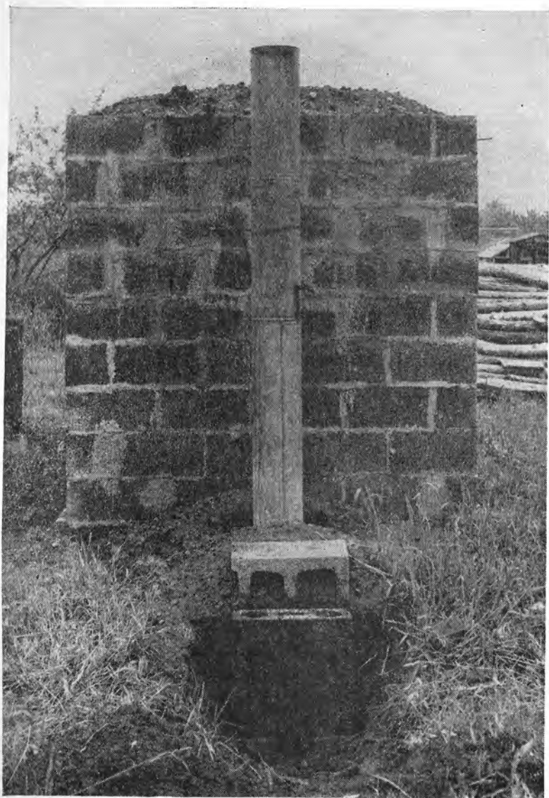
Front view of two-cord kiln with the chimney in place and the stove banked with earth except at the front end.
