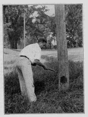
FIGURE 94. Method of injecting materials into poles with an "oil-gun".
