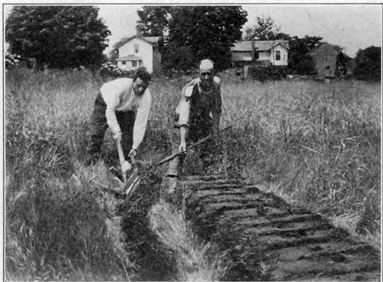
b. Removing the sod.
