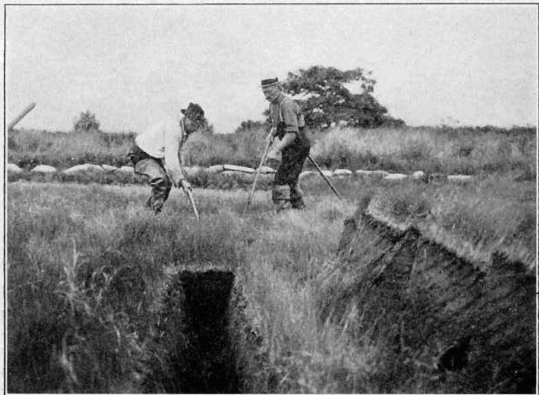
b. Cutting new ditch without special tools.
