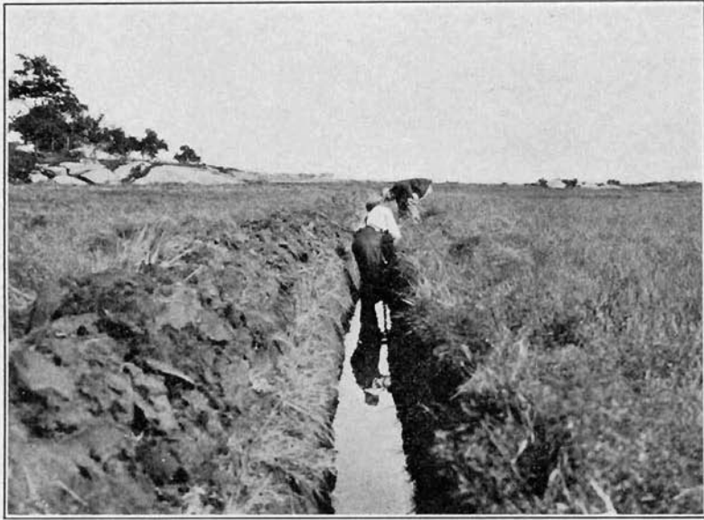
a. Cleaning old ditch.
