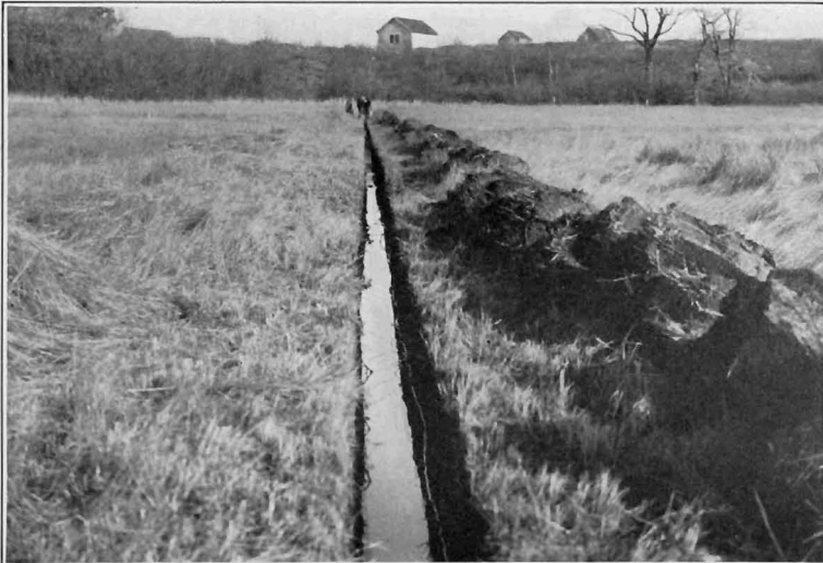
b. Hand cut ditch in salt marsh. MOSQUITO WORK, WESTBROOK.
