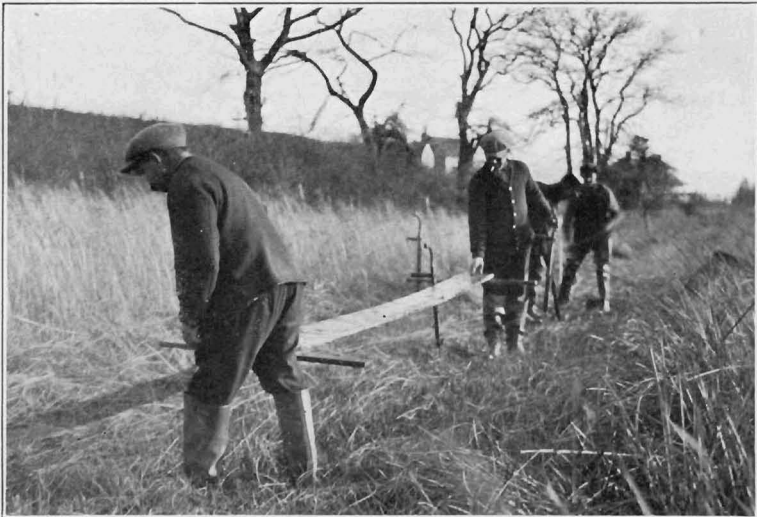
b. Guide board being placed in position for cutting ditch with hay knives.
