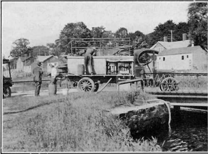
a. Automobile truck power sprayer taking water from canal.
