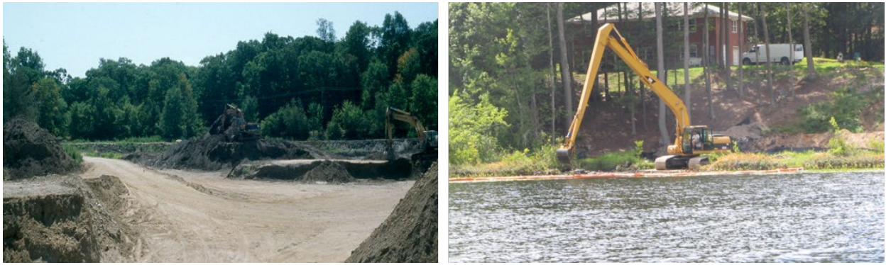
Figure 13. Dry dredging (left) and wet dredging (right)
