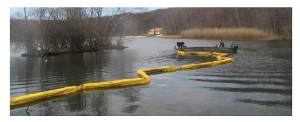
Figure 3. Installation of limnobarrier around island in Crystal Lake.
