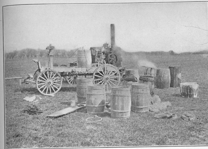
a. Cooking the lime, sulphur and salt mixture at Southington. A Kinney "Safe" engine furnishes steam to boil the mixture in barrels.
