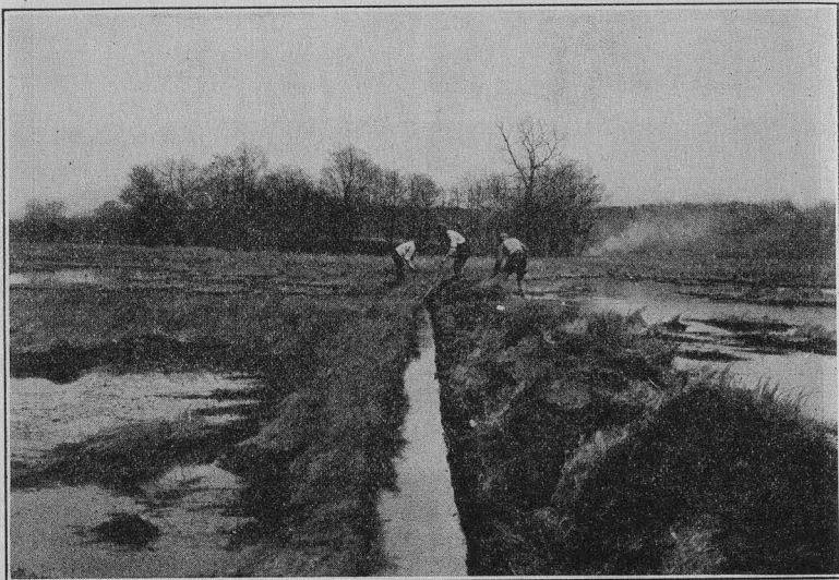
FIG. 3.—Anti-mosquito Work—cleaning out an old ditch.
