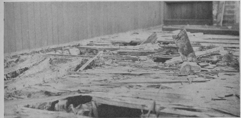
b. Rotten Condition of Living Room Floor.
