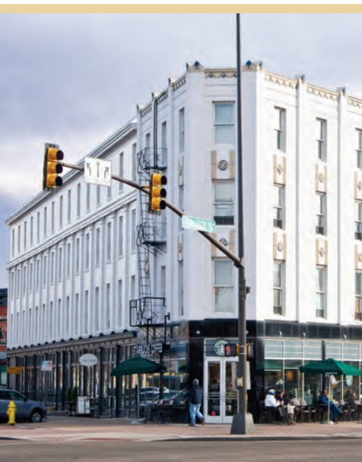
Northern Hotel rehabilitation in downtown Fort Collins, Colorado, historic district
