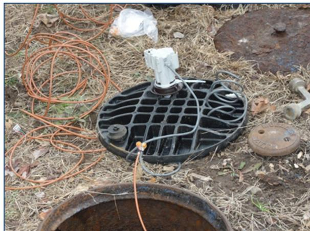
*MDC RF III – New Remote Reading Radio Frequency Device Attached to Underside of Meter Pit Cover*
