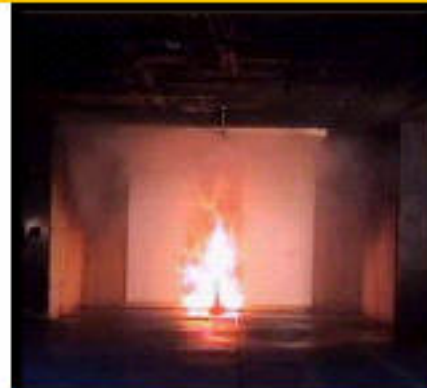
22 Seconds— Sprinkler Operates
