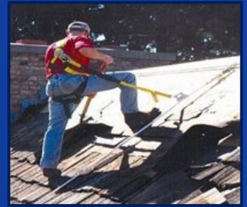
An example of a Personal Fall Arrest System in use during reroofing job duties
