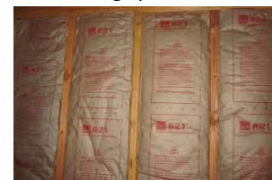
Fiberglass batts—vapor barrier correctly facing towards living space
