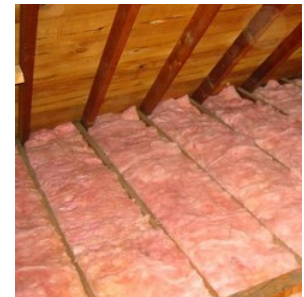
Fiberglass batts—vapor barrier correctly facing towards living space
