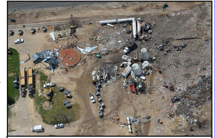
Aerial photo of the west explosion site taken several days after blast (4/22/2013). Photo credit: Shane Torgerson
