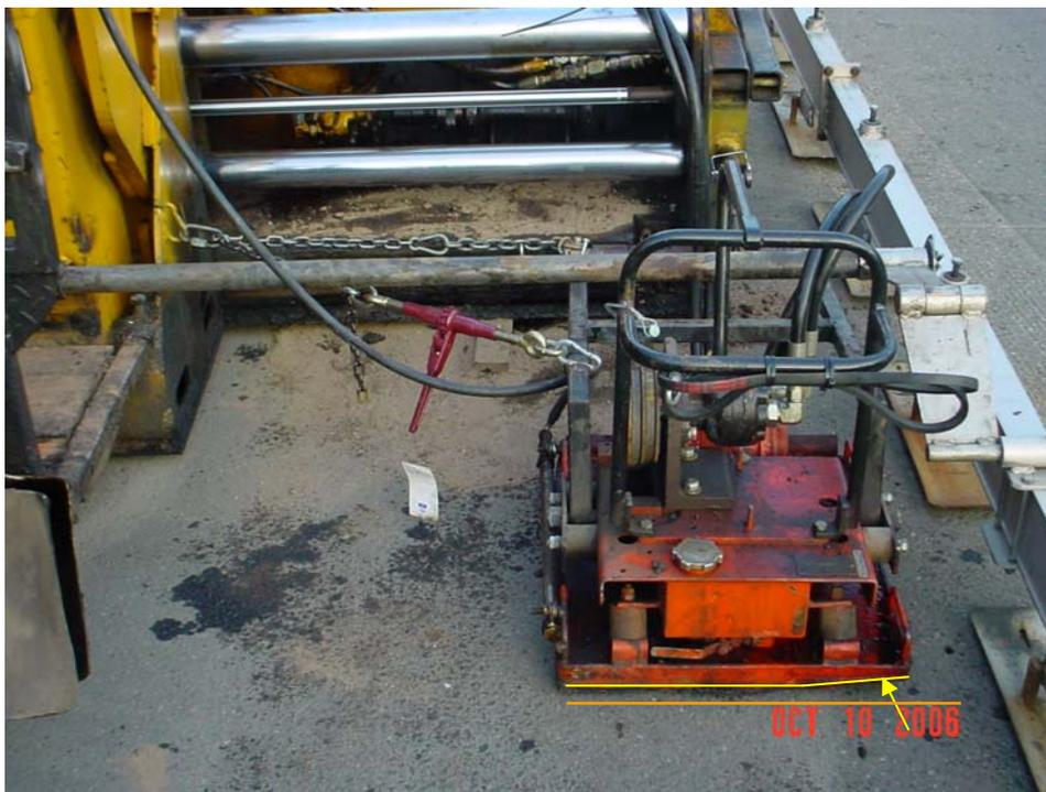
**Figure #3 Wedge Compaction Device and Setup**
