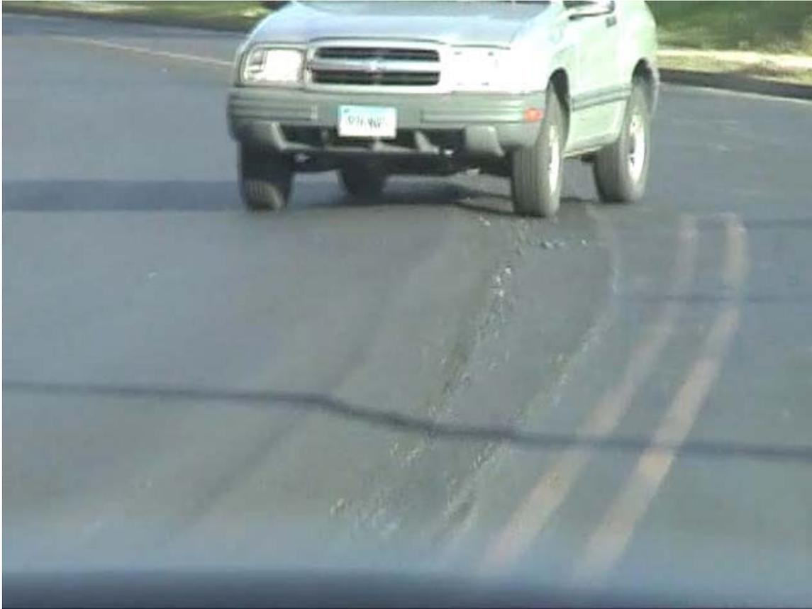
**Figure #8 Traffic Traversing Open Joint**
