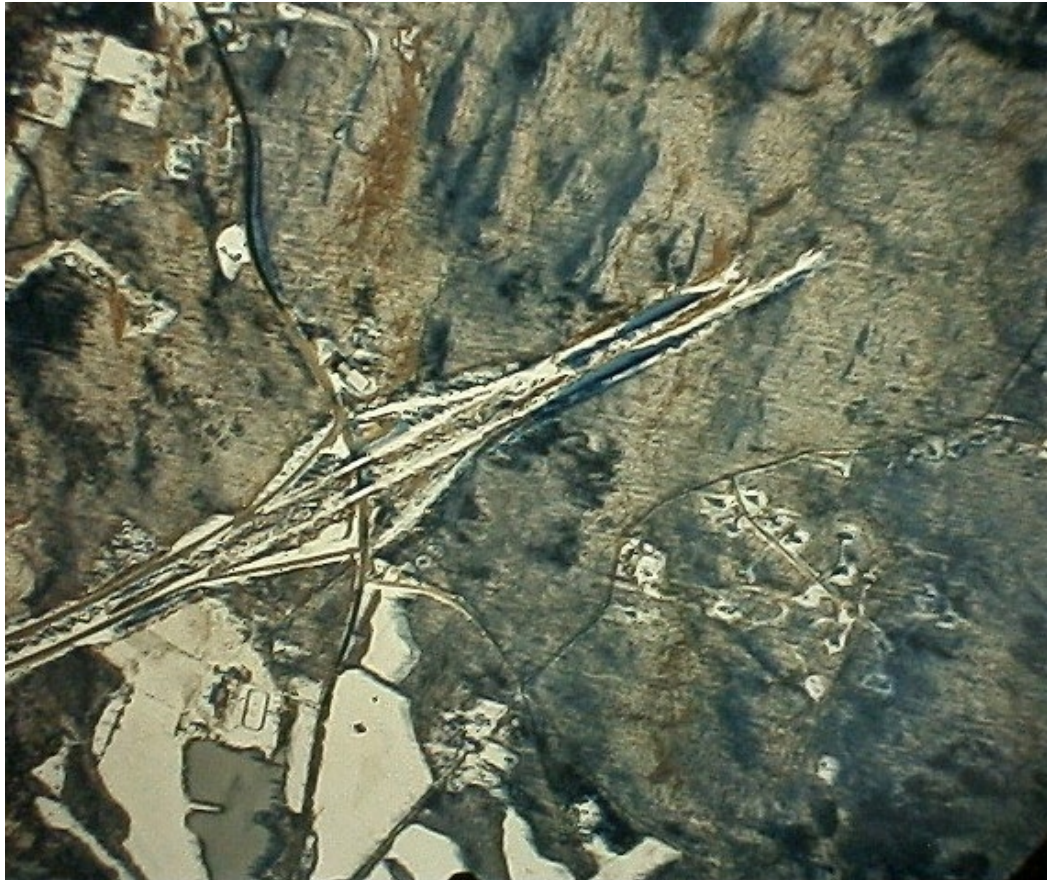
THIS AERIAL PHOTO, TAKEN IN NOVEMBER OF 1997, SHOWS THE TERMINUS OF ROUTE 11 AT ROUTE 82 IN SALEM. THIS VIEW CLEARLY SHOWS THE AREA THAT WAS PREPARED AND GRADED IN THE 1970S FOR CONTINUATION OF THE EXPRESSWAY TO I-95/I-395.
