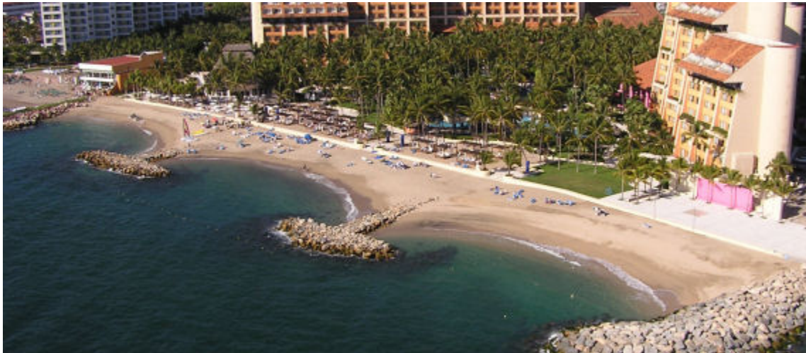
Figure 6 - Example of Offshore T-groins With Sand Deposit the Landward Side of the Beach
