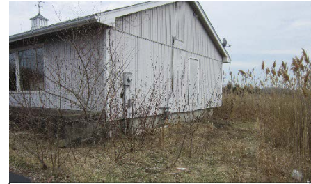
Utilities & adjacent wetland 26 Boston Post Road
