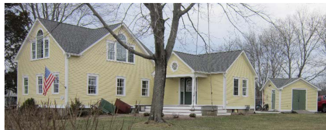
6 Old Post Road Note open bulkhead door
