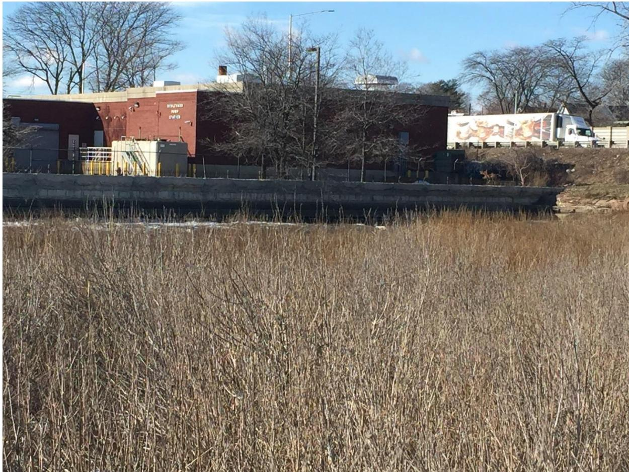
A view of the Pump Station located south of the Long Wharf Nature Preserve. Drainage channel from 36-inch stormwater outfall is present between the marsh and the Pump Station. The ground elevation around the Pump Station is about 10 feet NAVD88.
