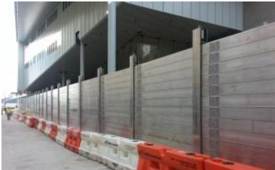
Examples of Aluminum Stop Log Flood Barrier
