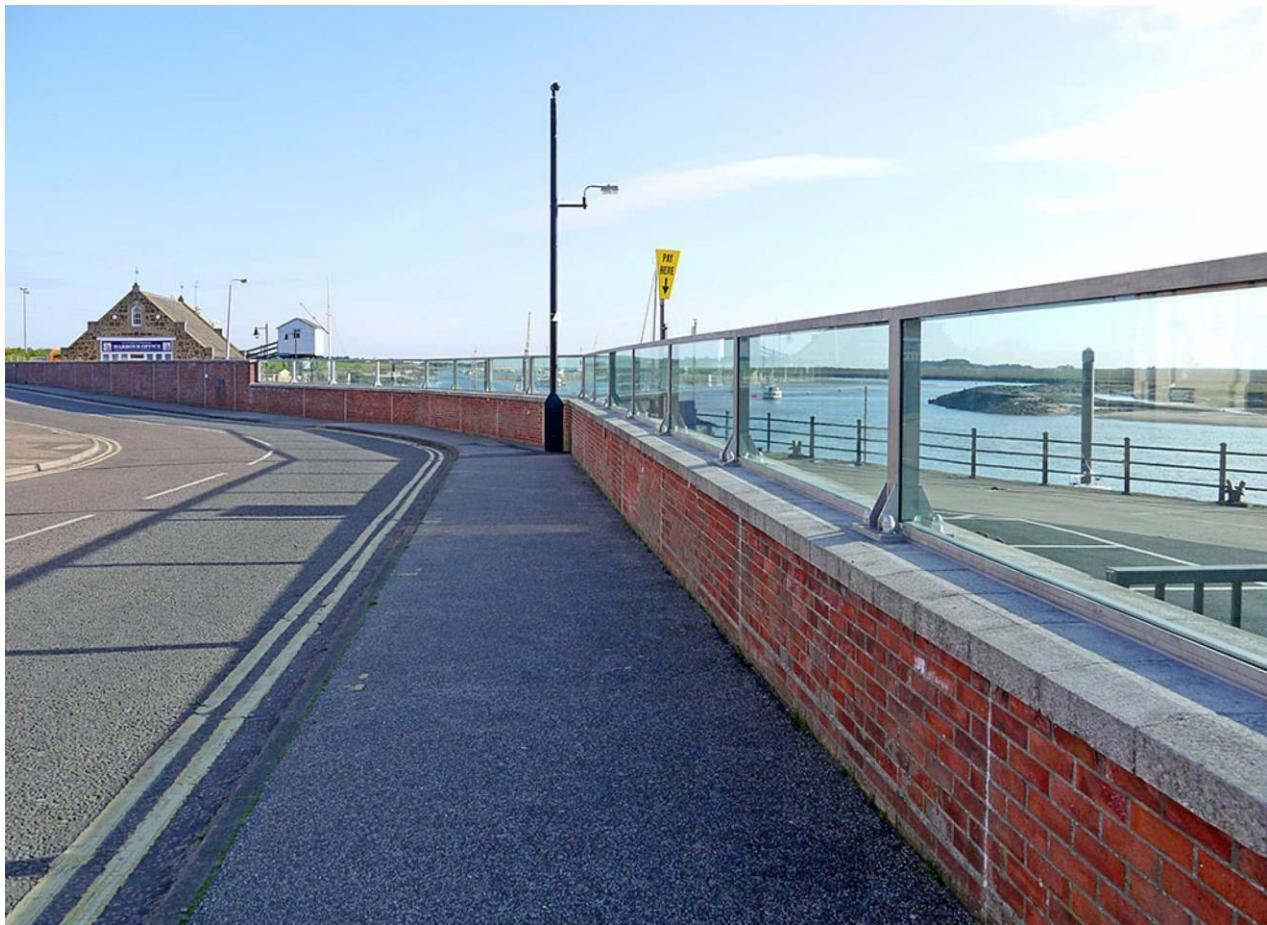
**Figure 6-15: Example of alternative flood wall design, with glass upper wall.**
