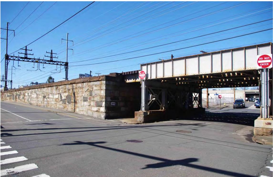
**Photograph 60. Railroad viaduct retaining walls, catenary structures, and the Myrtle Avenue Railroad Bridge, camera facing northwest.**
