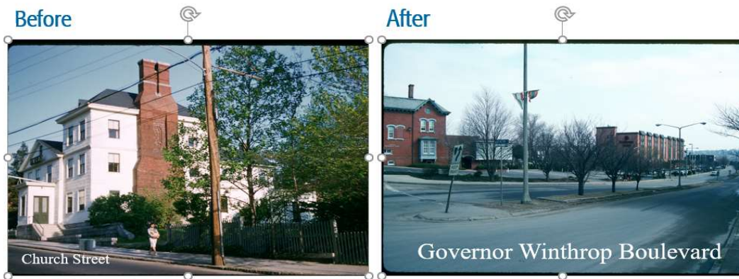
Figure 5 Photos of before and after urban renewal in New London, CT that show the widening of roads and demolishing of home. Photos accessed from the New London Landmarks, Inc.
