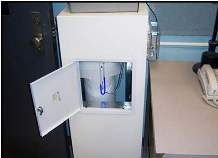
**One of the six Active Soil Depressurization units installed at the Garner Correctional Institution.**
