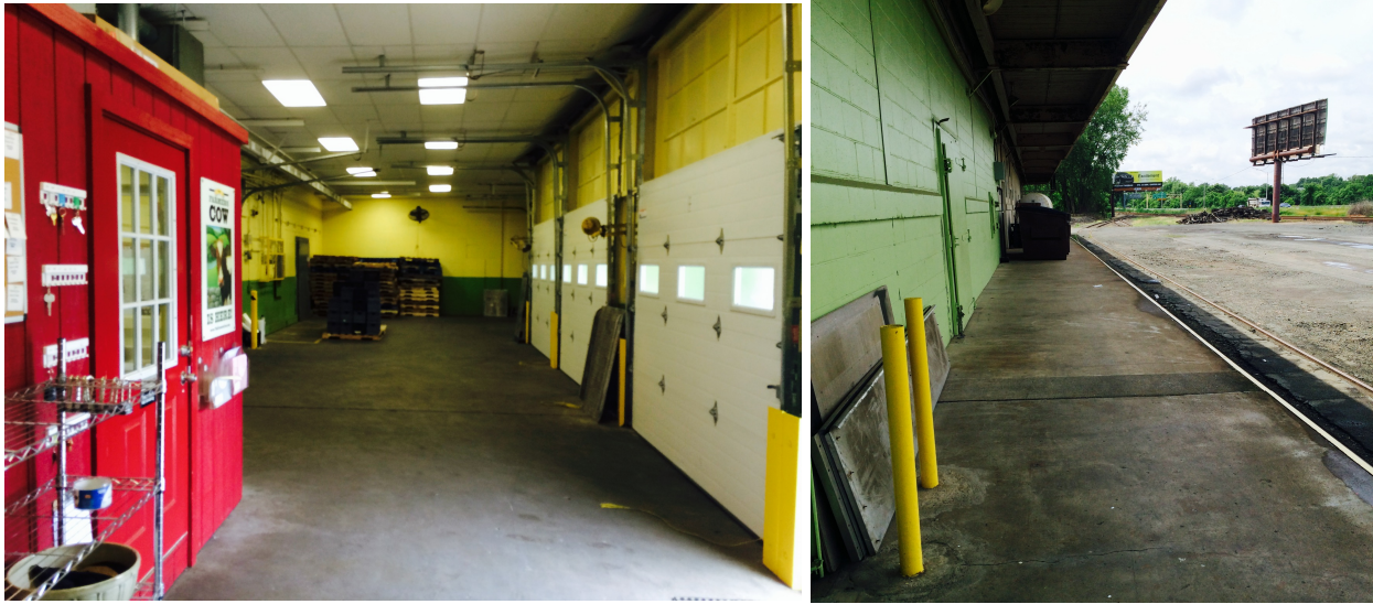
L- Interior of building, showing office and shipping and receiving area R- Exterior back of building, showing adjacency of rail spur
