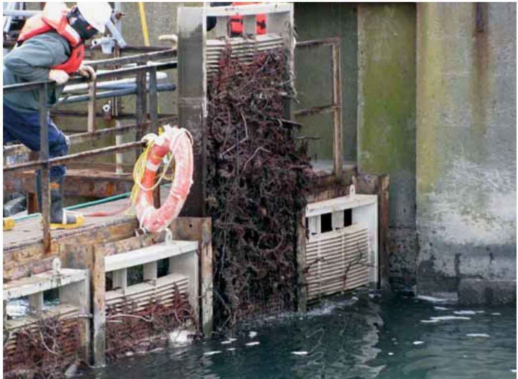
In January 2013, large amounts of HJ were found at Millstone Power Station in Waterford and carried through the power plant's cooling water systems. Extensive maintenance was required to remove all of this material from the intake and discharge structures.
