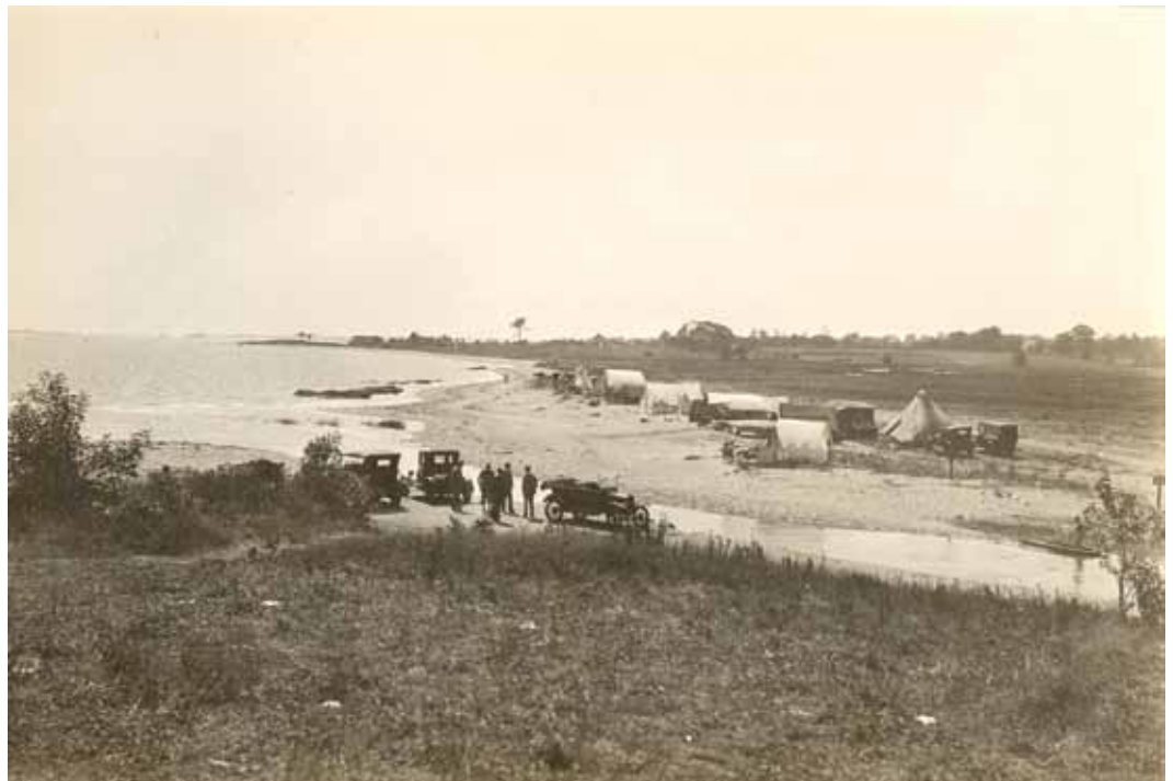
State Park Commissioners look across Westport's New Creek at the first five-acre land purchase at Sherwood Island. Although it was the first park property, the landlocked parcel had no official access until 1932. Until that time, illegal park users crossed the creek and encamped on the beach at their convenience.
