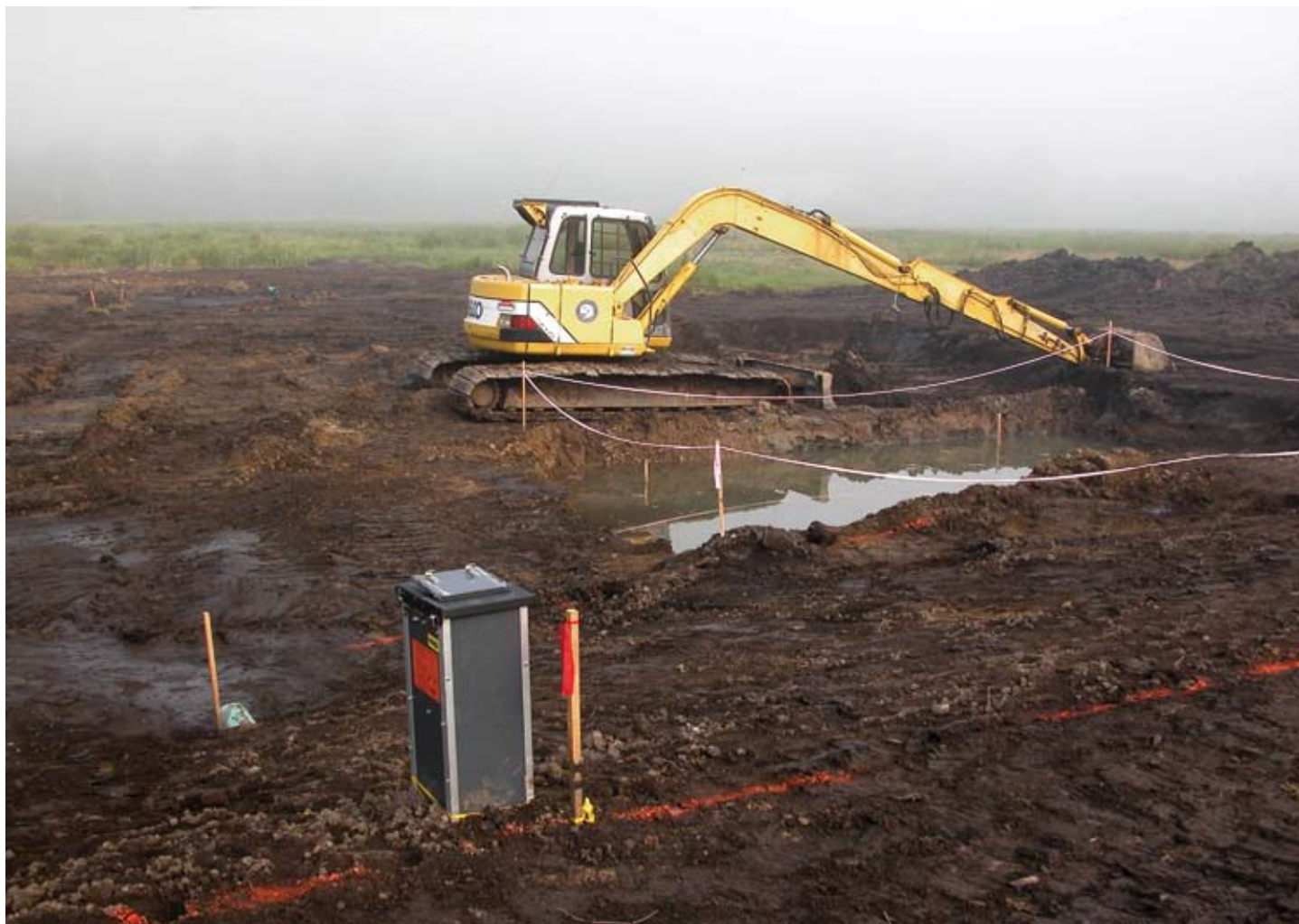
The WHAMM Program’s low ground pressure excavator is being used to construct a shallow water wetland. The water control structure in the foreground will be installed to control the water level.
