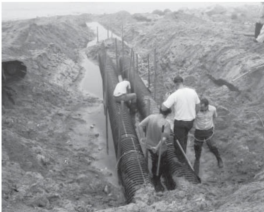
**Workers install two culverts in East Lyme to restore a tidal pond that had previously converted to a freshwater pond.**
