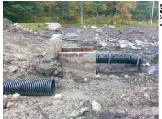
The old cement water control structure at Pumpkin Hill WMA with two plastic pipes.
