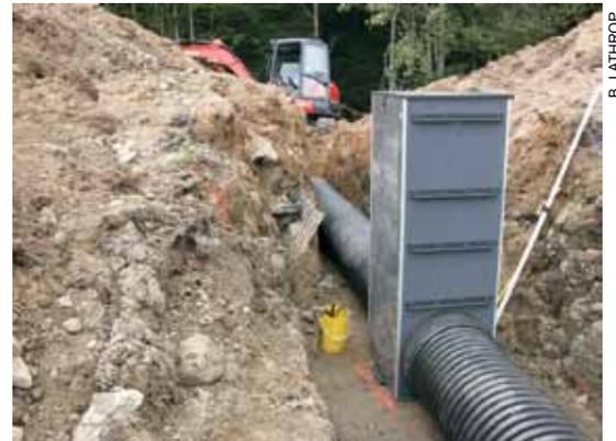
View of a 24-inch diameter ADS N-12 pipe attached to an eight-foot Agri-Drain inline water control structure.
