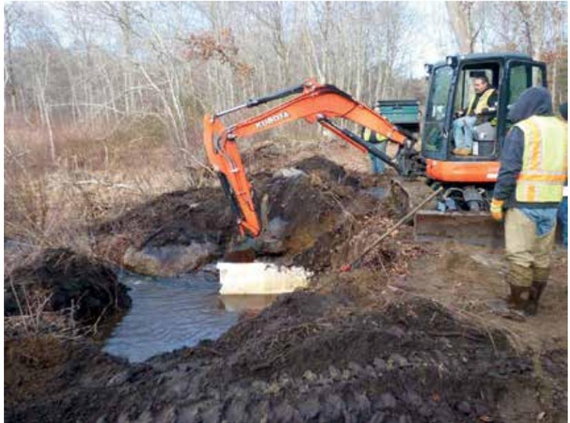
Steve Rosa, with the Wildlife Division's WHAMM Program, uses an excavator to remove a small amount of material from the existing culvert in preparation for the installation of the water control structure.
