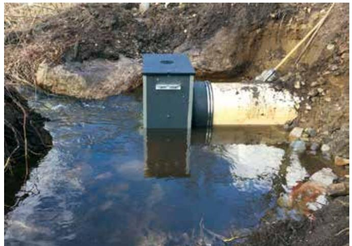
Weir boards within the water control structure will be adjusted at certain times of the year to optimize water levels for various wildlife species.
