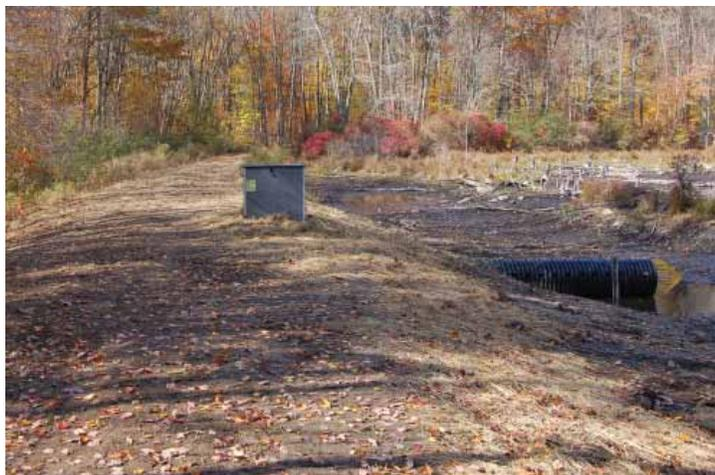
**(Top)** DEP Wetlands Habitat and Mosquito Management Program staff installing an in-line design water control structure at Bartlett Brook WMA in Lebanon. **(Bottom)** This device allows the Wildlife Division to manage water levels at suitable depths for wetland dependent species. It also minimizes water flow impacts by nuisance beaver.
