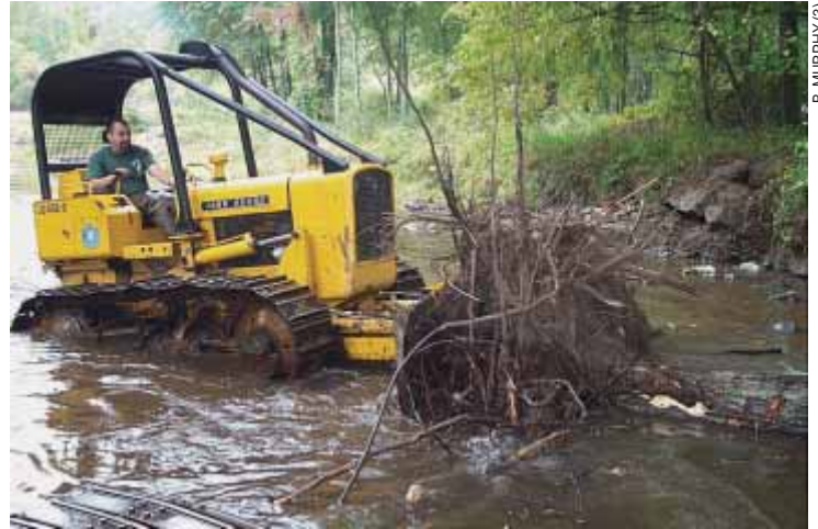
A bulldozer moves a root ball into position in the river bank. Root balls were installed to further deflect stream flow away from streambanks and to provide refuges for fish.
