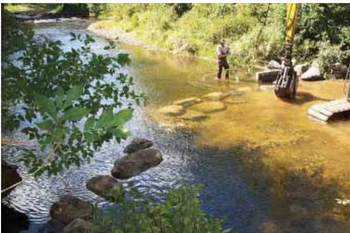
The excavator also was used to build a weir dam with rocks. A weir dam maintains pool habitat and concentrates stream flows toward the center of the channel, away from eroding streambanks.
