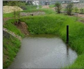
Generally porous asphalt performs well for those chemicals relating solid concentrations. Retention ponds also remove solids but achieve greater removal of DIN as well. Dissolved contaminants are more difficult to remove. Nitrogen is regulated off the dissolved portion. Metals are only regulated in their total concentration, while much lower in concentration, the dissolved portion often represents the more toxic form.
