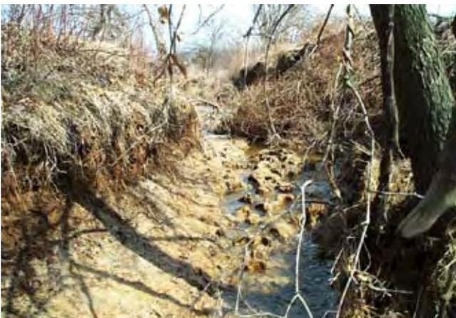
**Figure 2-12** Local instability problem above a township bridge. This channel became misaligned with the bridge opening due to lateral migration. The treatment includes stream barbs and a rock riffle grade control structure to protect against possible degradation as a result of shortening the channel during realignment. (Bay Creek, Pike County, IL)
