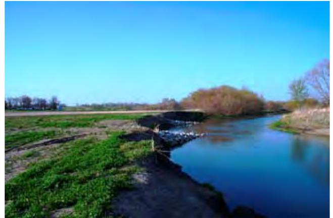
(c) September 2001—10 months after installation of stream barbs. Eroding banks have sloughed to stable angle and revegetated.
