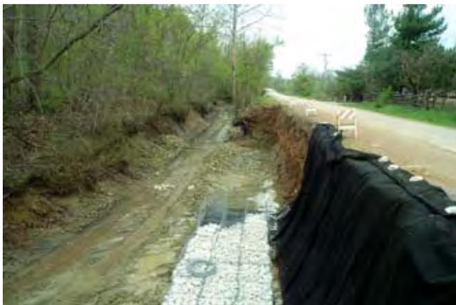
(b) June 2003—2 months after treatment using rock riffle grade control structures to stabilize bed and gabion baskets to stabilize failing bank near road. Note water impounded in pool.
