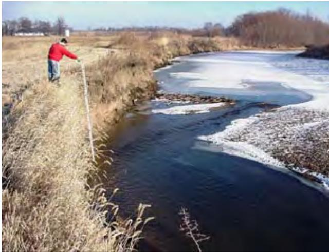
(b) April, 2001—5 months after installation of stream barbs. No shaping or seeding of banks was included in project. Eroding banks will be allowed to vegetate naturally.
