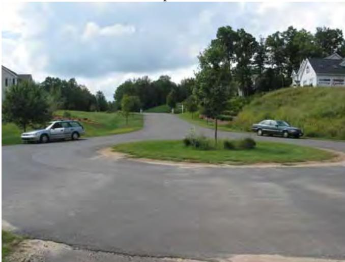
**Source:** CT NEMO LID Inventory - Site with reduce road widths, no curbing, vegetated infiltration island and pervious pavement
