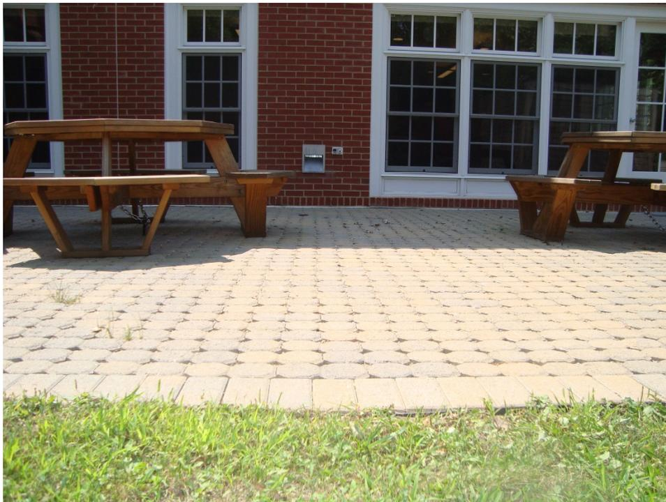
**Figure 9. Pervious pavers at Lakeside Apartments.**
