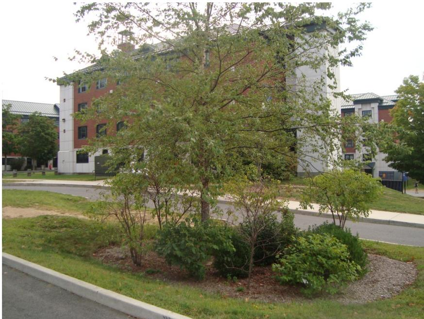
**Figure 5. Bioretention by Towers dorms.**
